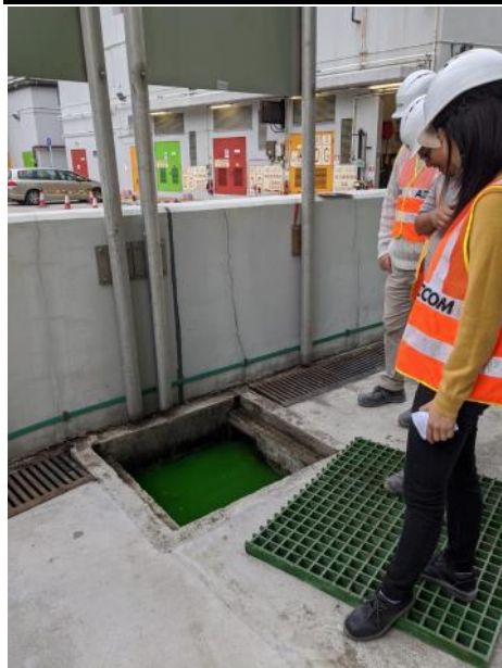
Figure.5 Dye test carried out on 30 December to ensure the gate valve is fully closed
